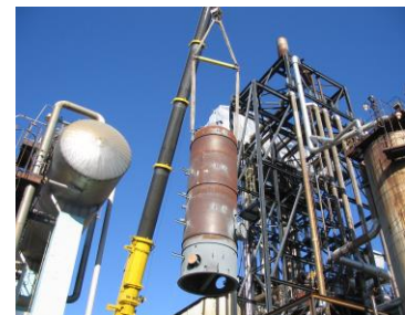
Vessel fabrication & Installation.
